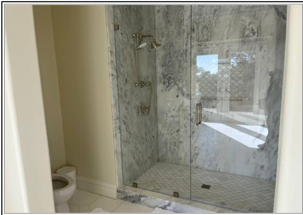
Interior Photo Bathroom
