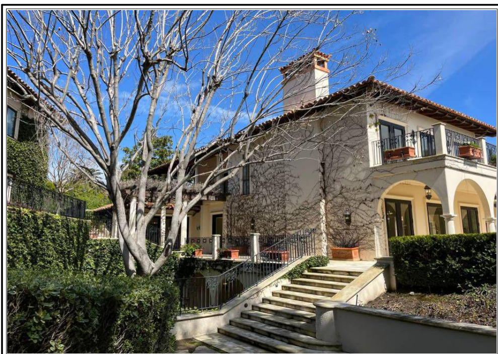
Exterior Photo Side
