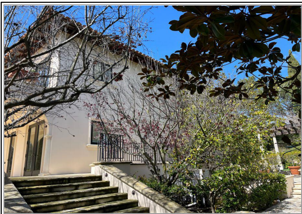
Exterior Photo Side
