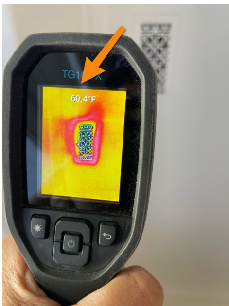
Example Noted At Master Bedroom Closet
