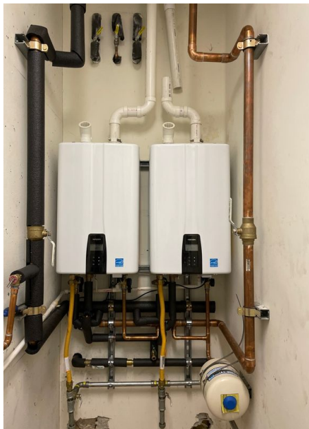
Example Noted At Basement
