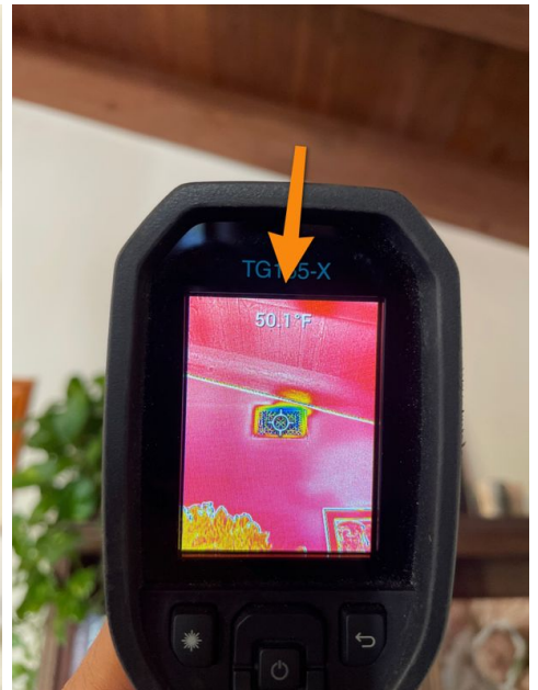
Example Noted At pool House
