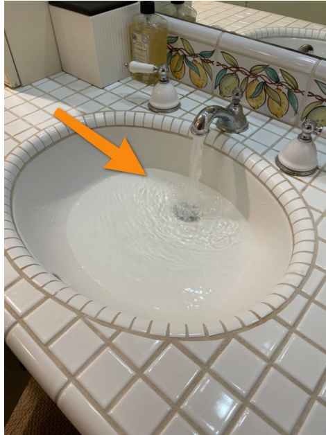
Example Noted At Pool House Bathroom
