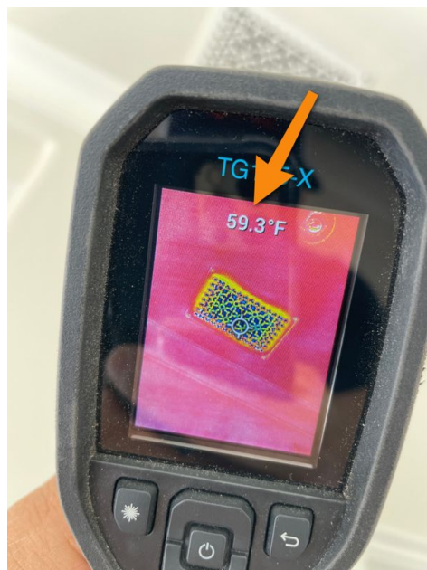
Example Noted At Bedroom 4
