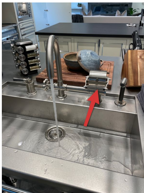
Example Noted At Kitchen
