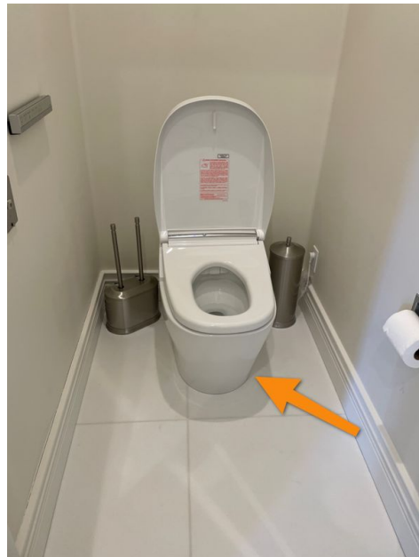
Example Noted At Master Bathroom
