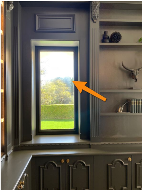
Example Noted At Office
