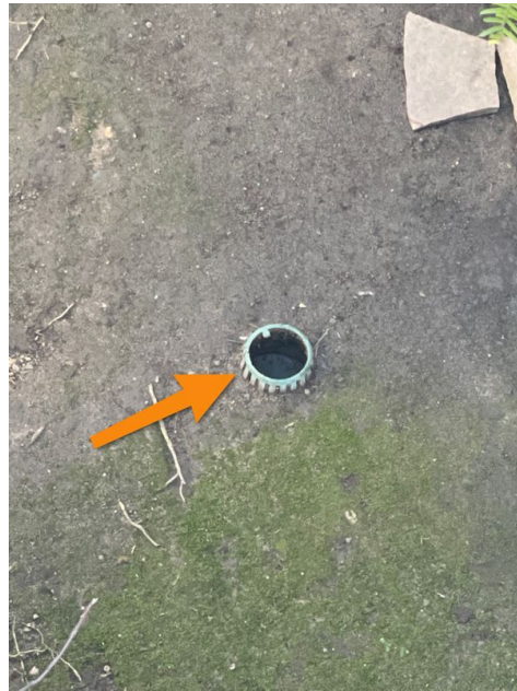
Example Noted At Left Side Of Home
