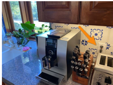
Example Noted At Pool House Kitchen
