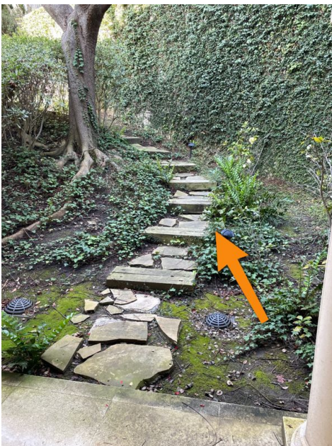
Example Noted At Right Side Of Home
