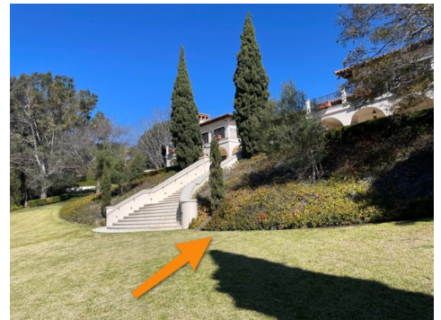
Example Noted At Rear Side Of Home
