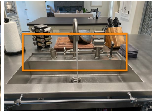
Example Noted At Kitchen
