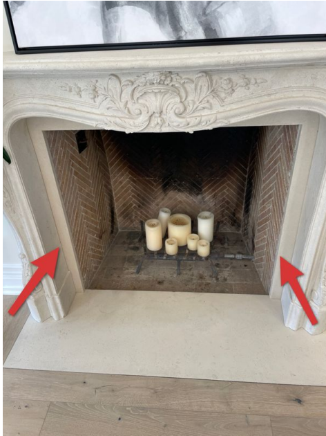
Example Noted At Dining Room
