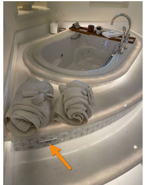
Example Noted At Master Bathroom
