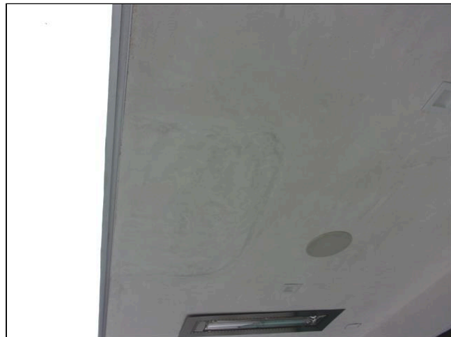
Repair To Exterior
