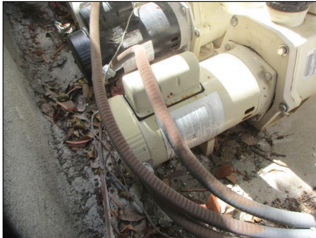
Pumps Not Bonded To Ground
