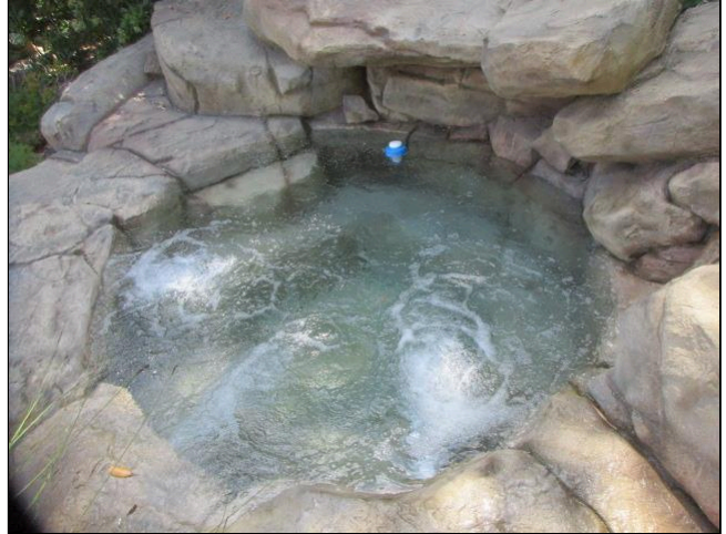
Spa Booster Pump Not Operating Properly
