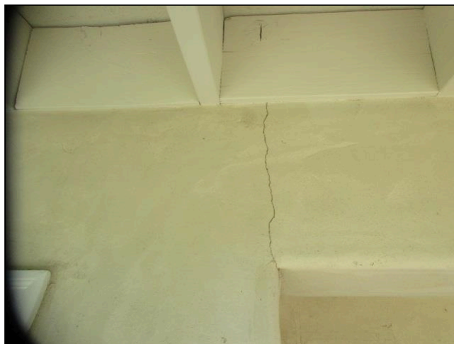
Stucco Cracks
