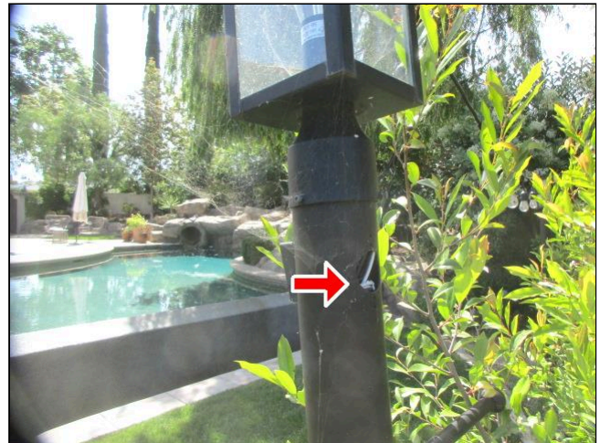
Exposed Wiring
