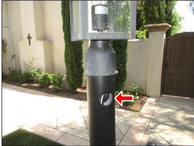
Exposed Wiring
