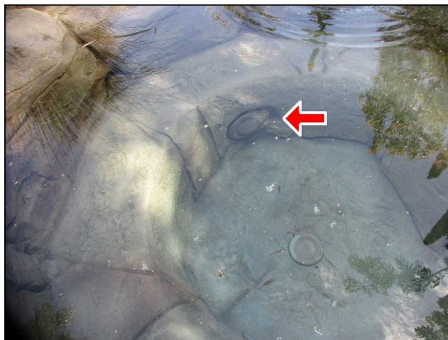
Spa Light Not Operational
