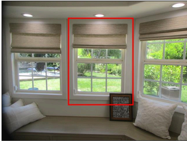
Faulty Channel Balance
