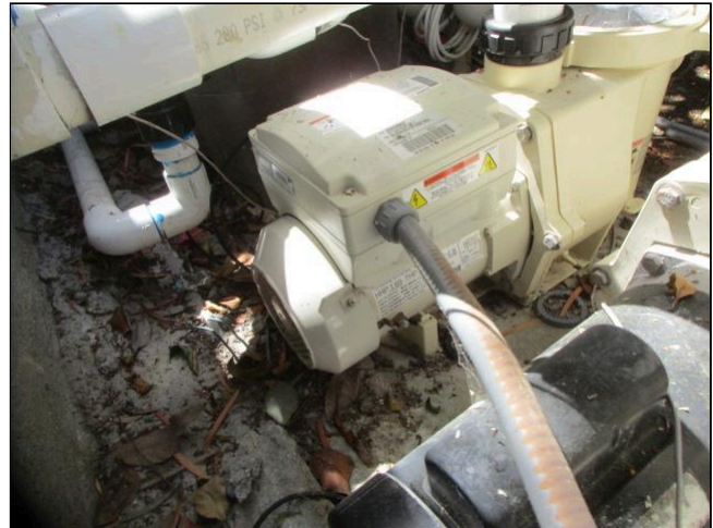
Pumps Not Bonded To Ground
