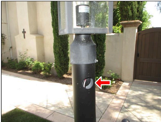
Exposed Wiring
