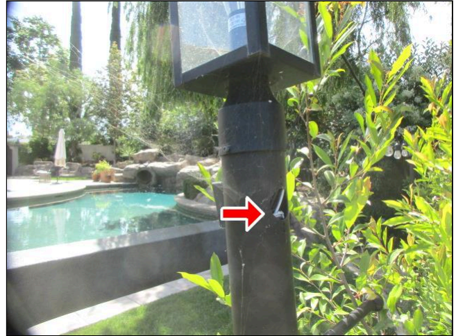
Exposed Wiring
